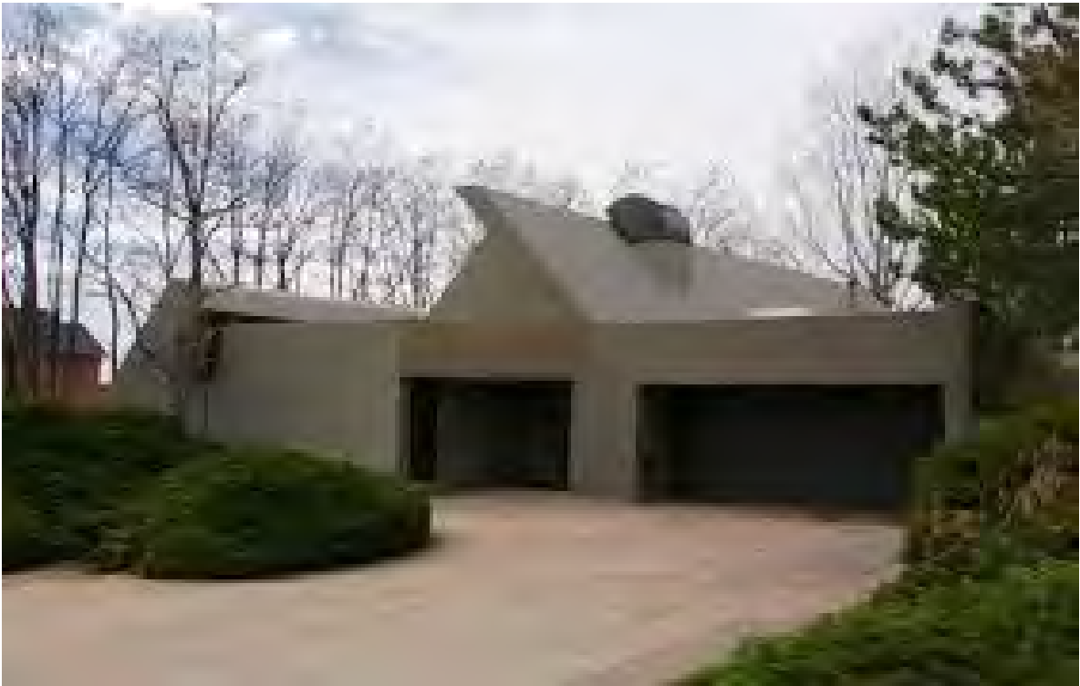
Photo 65: Richard Crowther's Cherry Creek home, demolished 2024
