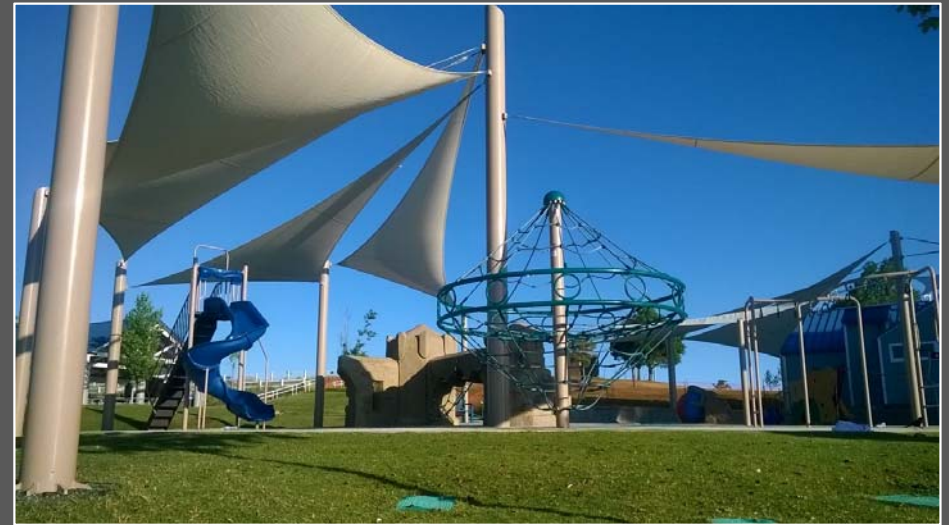
Playground Shade Shelter
