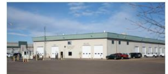
Central Facility Administration Building and Shop Building, including Fleet Maintenance
