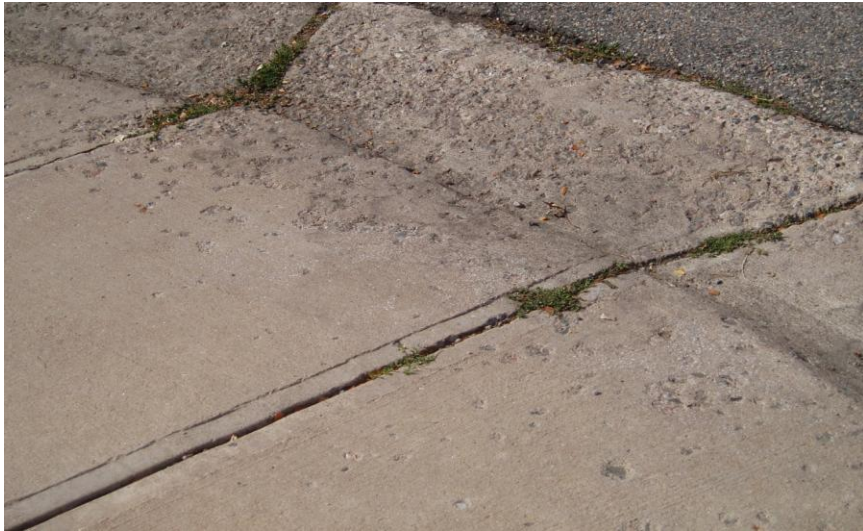
MODERATE SPALLED
