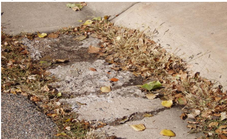
SEVERE SPALLED
