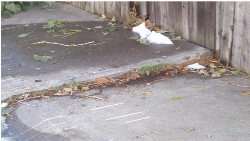
SEVERE DISPLACEMENT
