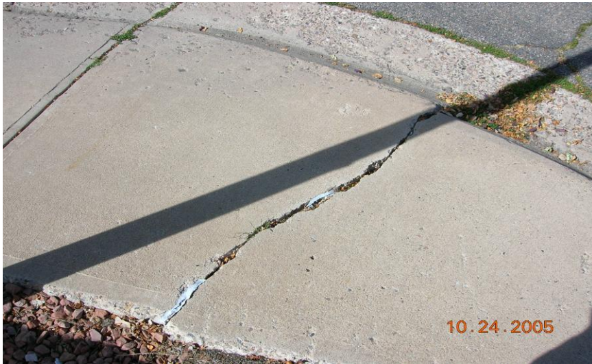
MODERATE CRACK
