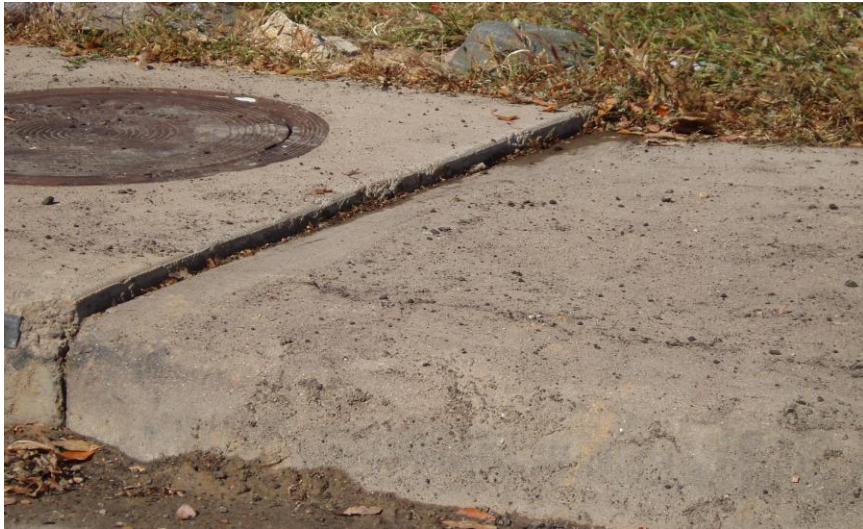
MODERATE DISPLACEMENT
