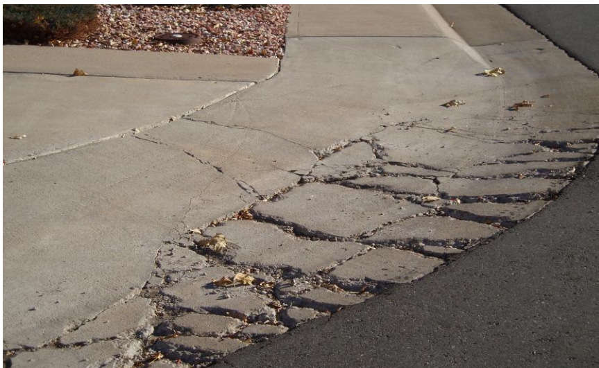
SEVERE CRACK
